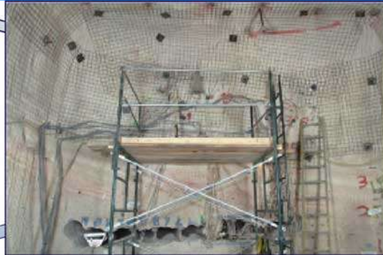
(a) Photograph of Alcove 4 Test Bed
