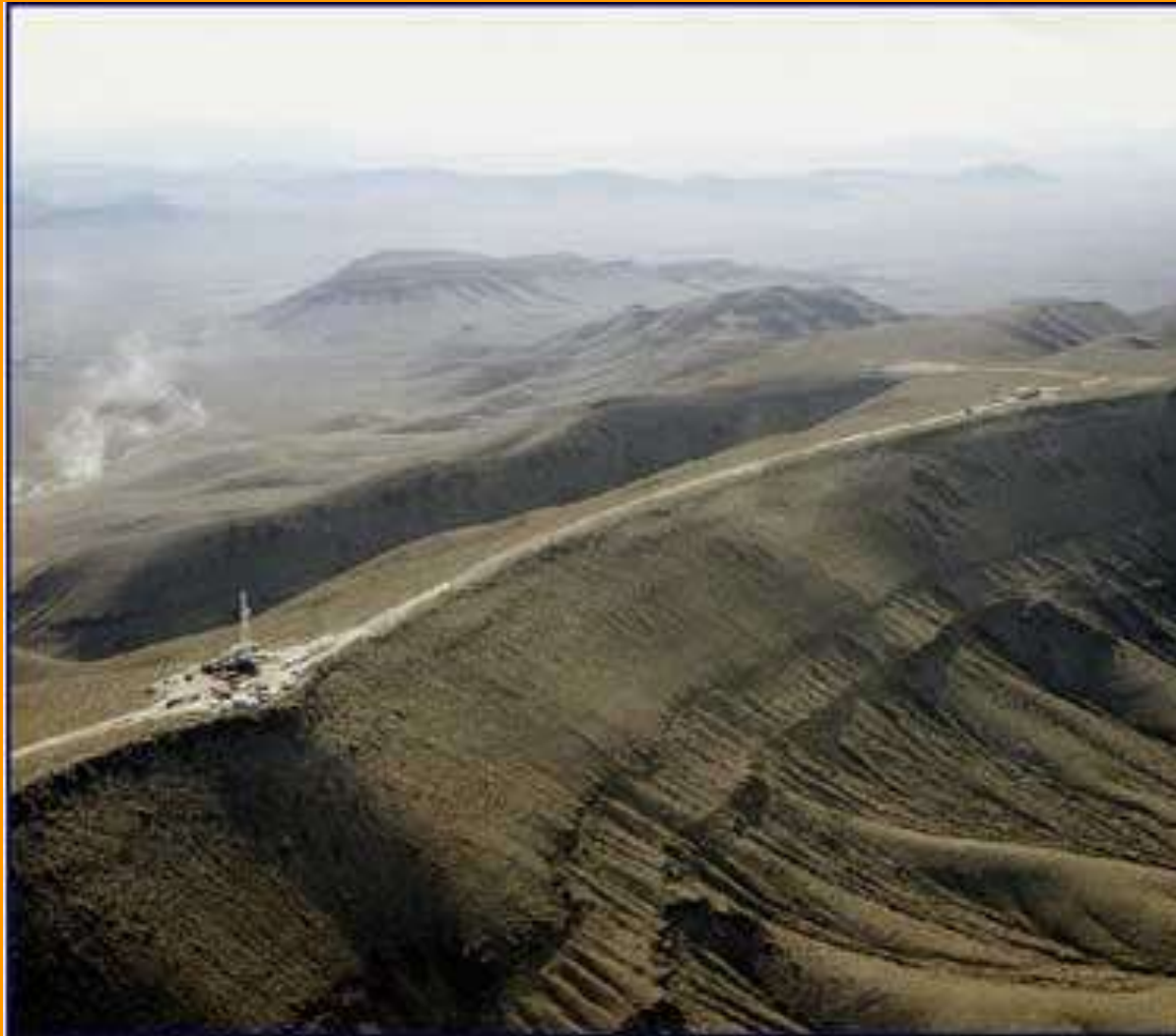
(a) Drilling of Borehole SD-6 on the Crest of Yucca Mountain
